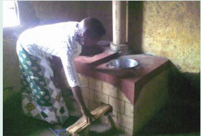
Photo 19: A woman cooking with an improved wood fuel stove built in Kilimanjaro region.
