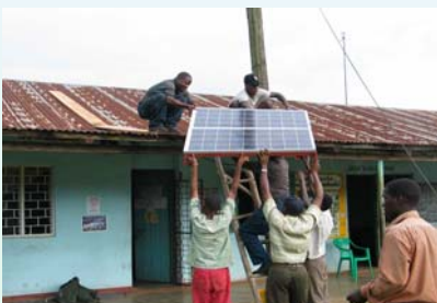
Solar PV installation
