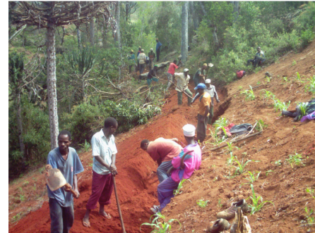
Villagers' participation during excavation canal headrace
