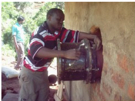
TaTEDO Engineer installing mechanical joint for holding the penstock
