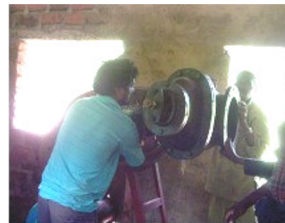
UNIDO Consultant installing control sluice valve
